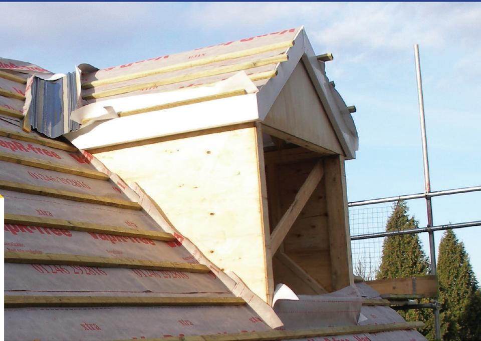
*VapR-free Xtra* is a multi layer laminate film composite made of polyolefin materials, resulting in a pitched roof underlay that has high vapour permeability, but is also highly water resistant.
